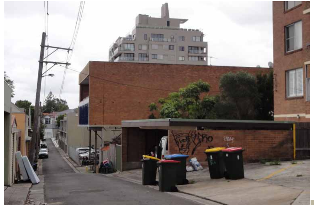
Chesterfield Lane streetscape - view towards site from east
