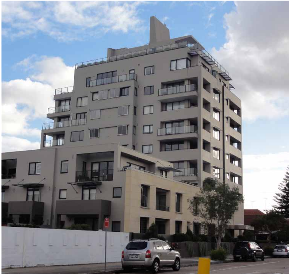
The Ocean View apartments building - Macpherson Street frontage
