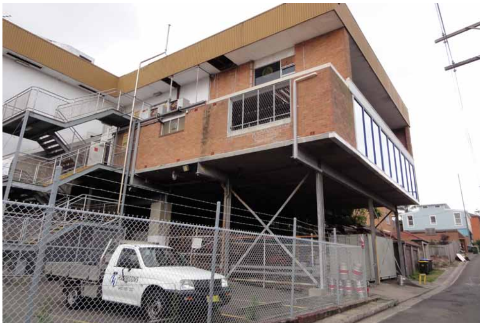
The existing building facing Chesterfield Lane
