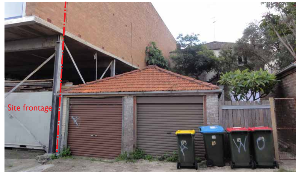
Relationship between site (left) and 119 Macpherson St. to east (right) along Chesterfield Lane
