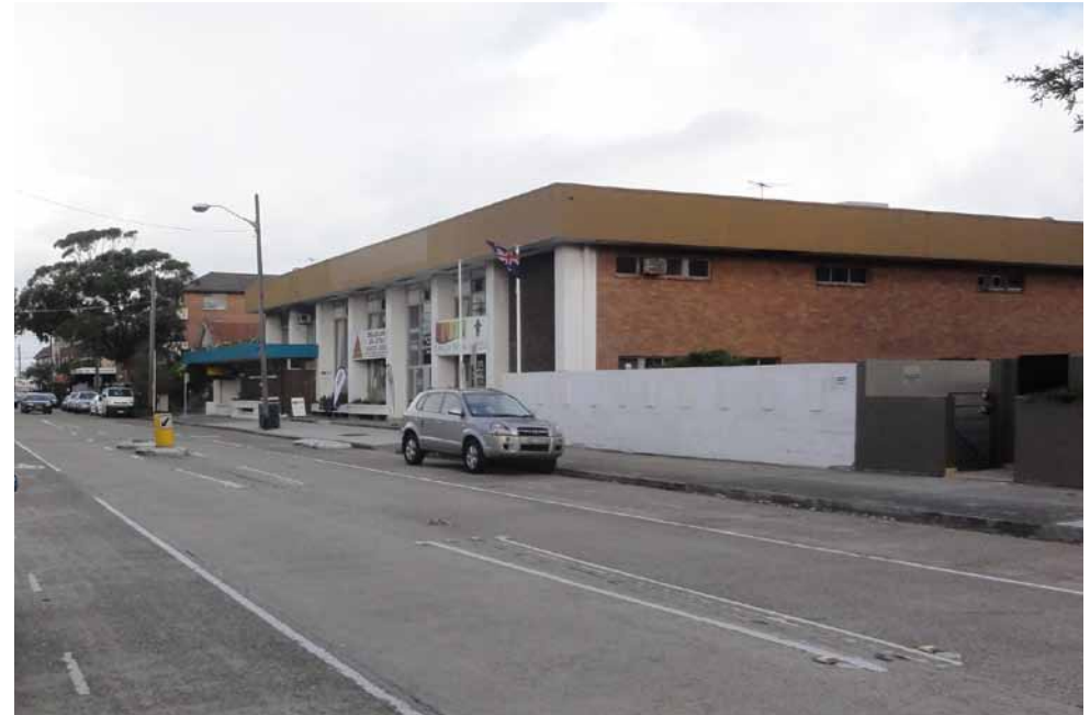
The Macpherson Street frontage of the site and the existing building
